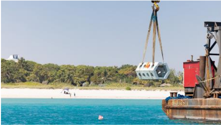
SEAHIVE unit being lowered into the ocean off Surfside, Miami Beach
