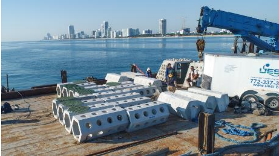
Hybrid reef structures on barge prior to deployment
